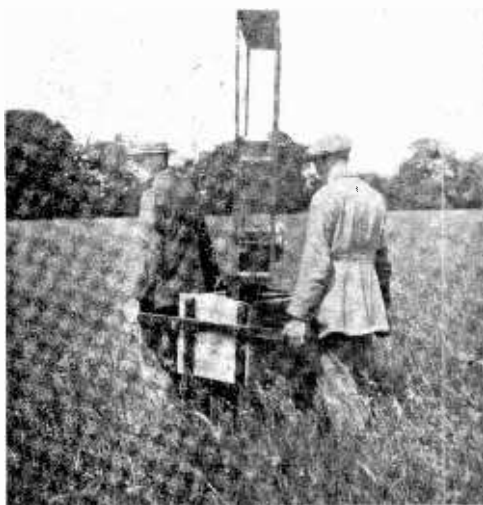
Fig. 4a. Photograph showing mode of carrying the D.F. set without dismantling.
