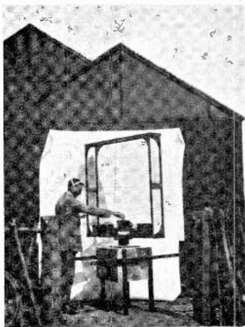
Fig. 5c. Portable single-frame direction finding set.
